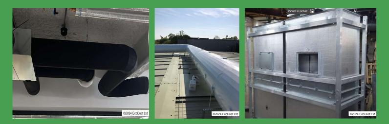
EcoDuct can be used anywhere where insulated ductwork is required – primary supply and return air, FCU discharge/secondary, plant room, risers, external ductwork, etc. EcoDuct is available in any size, shape and colour finish.
